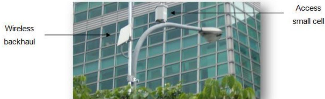
**Figure 4: Sub 6 GHz Deployment on a Lamppost**
