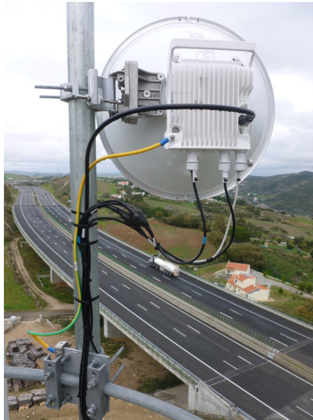
FibeAir IP-20C can be remotely upgraded from 1+0 to 2+0, doubling capacity without site visits
