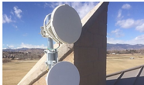
Siklu links boost urban anchors capacity in the City of Arvada, Colo. from 1.5Mb to 1Gb. An increase of 70 times the throughput
